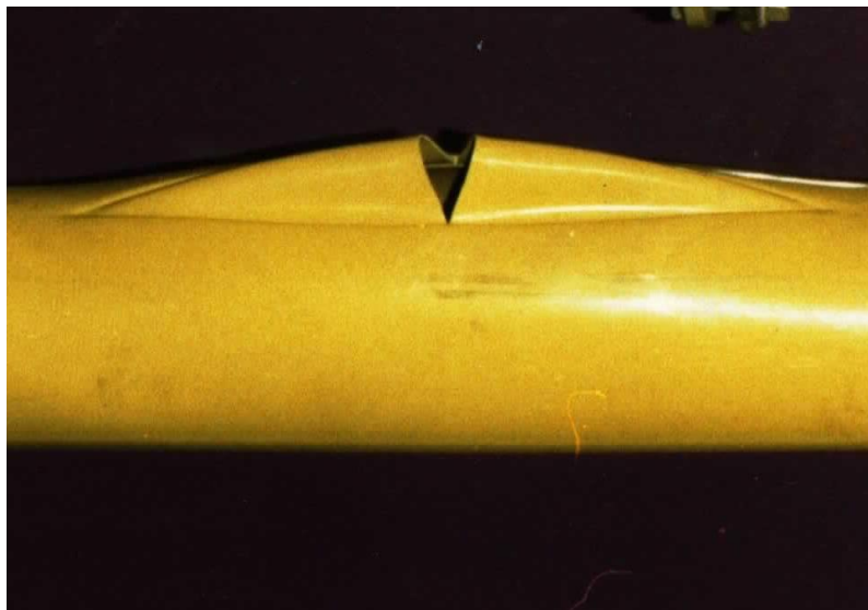
Figure 3 Ductile Failure of PE Pipe Under Internal Hydrostatic Pressure
