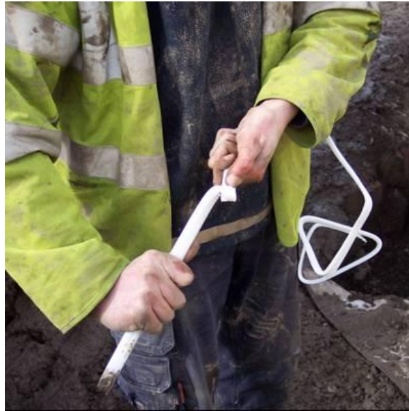
Figure 15 Bead Quality Control (Bend Back Test)
